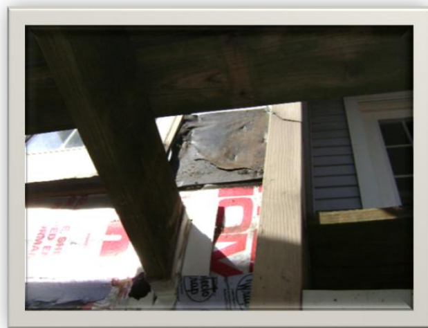
The black rubber flashing was never unfolded.
